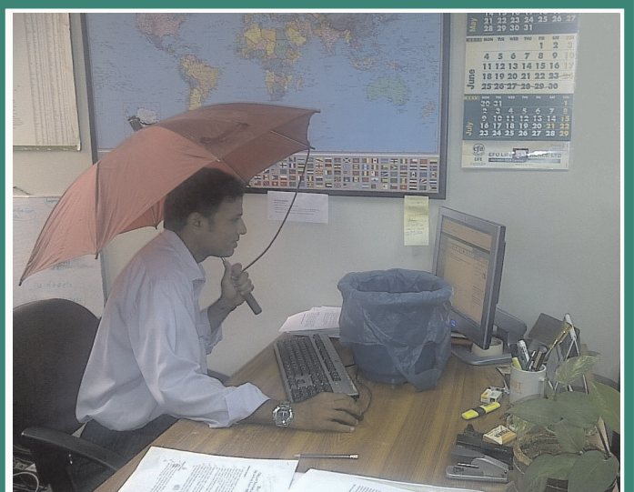
It takes more than a small roof leak to stop work in CBEC! With a strategically placed bucket on his desk, and an umbrella positioned over his head Aamir Shehzad, CBEC's IT staff, calmly continues his work.
